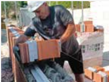
POSA IN OPERA
