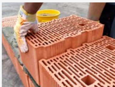
POSA IN OPERA
