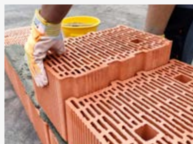
POSA IN OPERA
